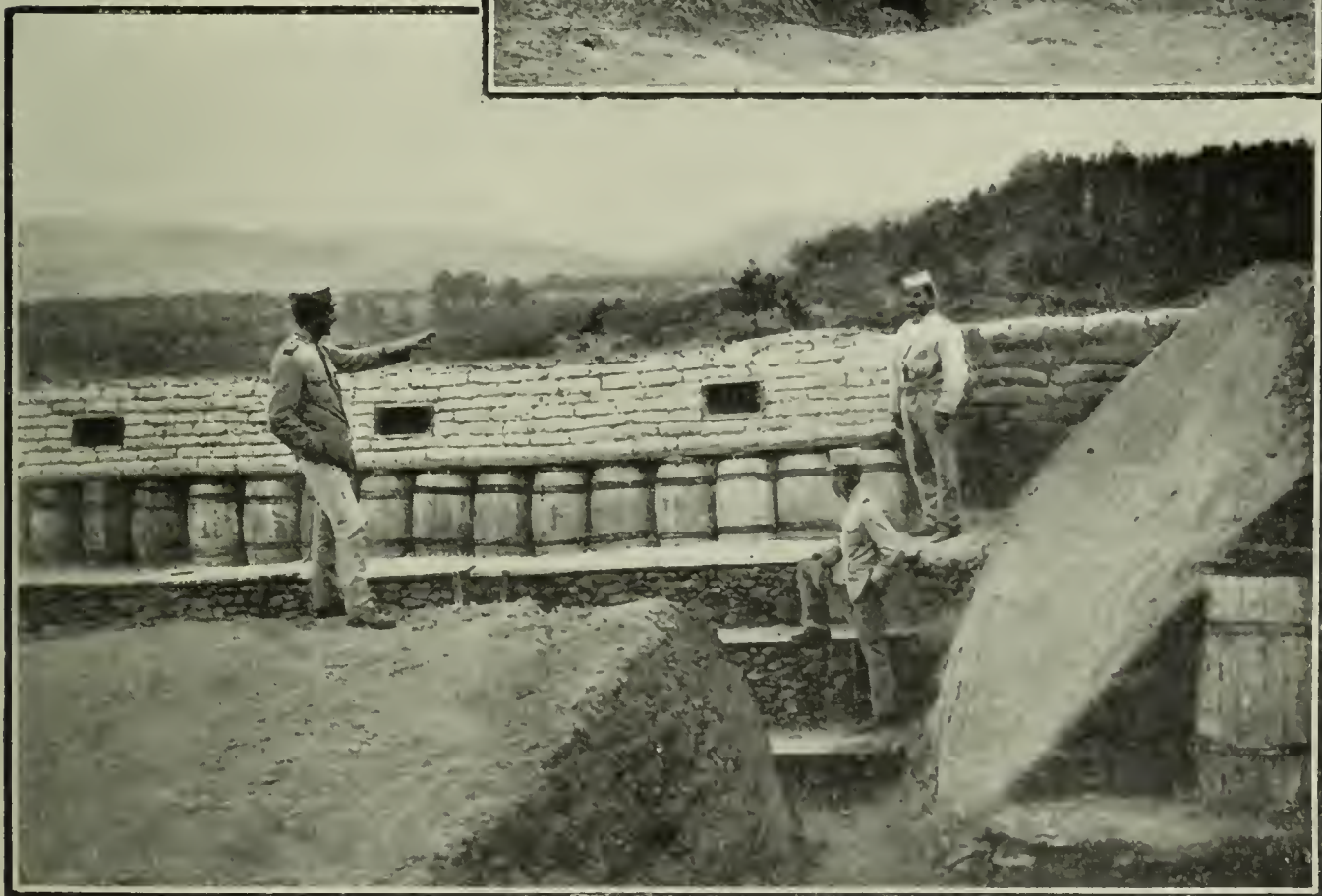
Sappers preparing a trench.
