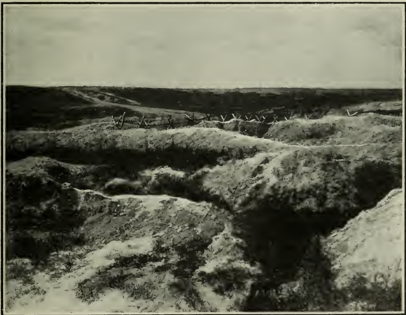
AUSTRIAN TRENCHES AND DUG-OUTS Captured by the Russians
