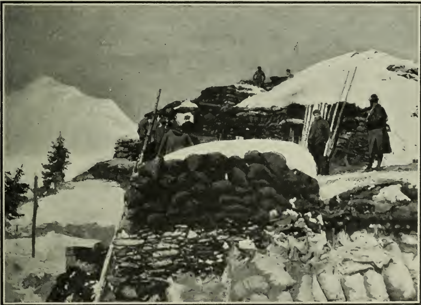
AN ITALIAN TRENCH IN THE MOUNTAINS. 2,000 metres high.
