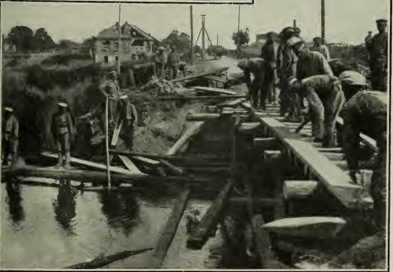
Russian engineers repairing bridges destroyed by the Austrians. Centre picture: Russian Cavalry crossing a hastily built bridge.
