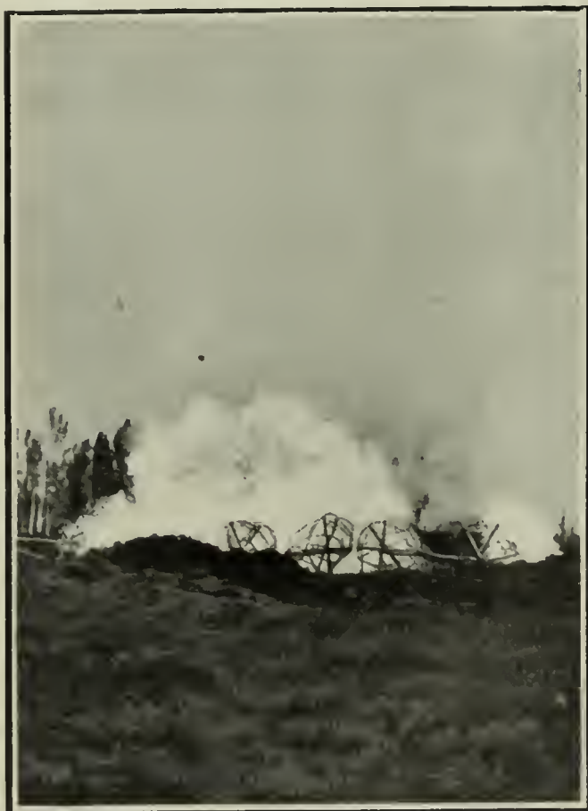
Explosion of the tube, causing destruction of an Austrian trench.
